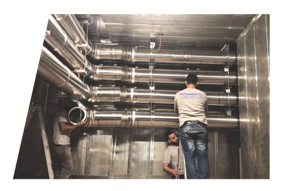
• Fittings include various angle elbows, tees, adaptors, soot collectors, and terminal caps, as well as a variety of structural accessories needed for support and attachment to building structures.
